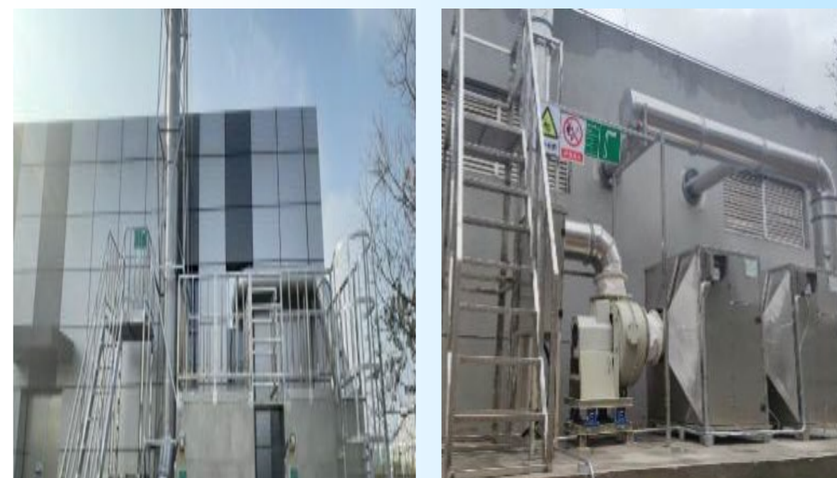
Waste gas treatment facility
